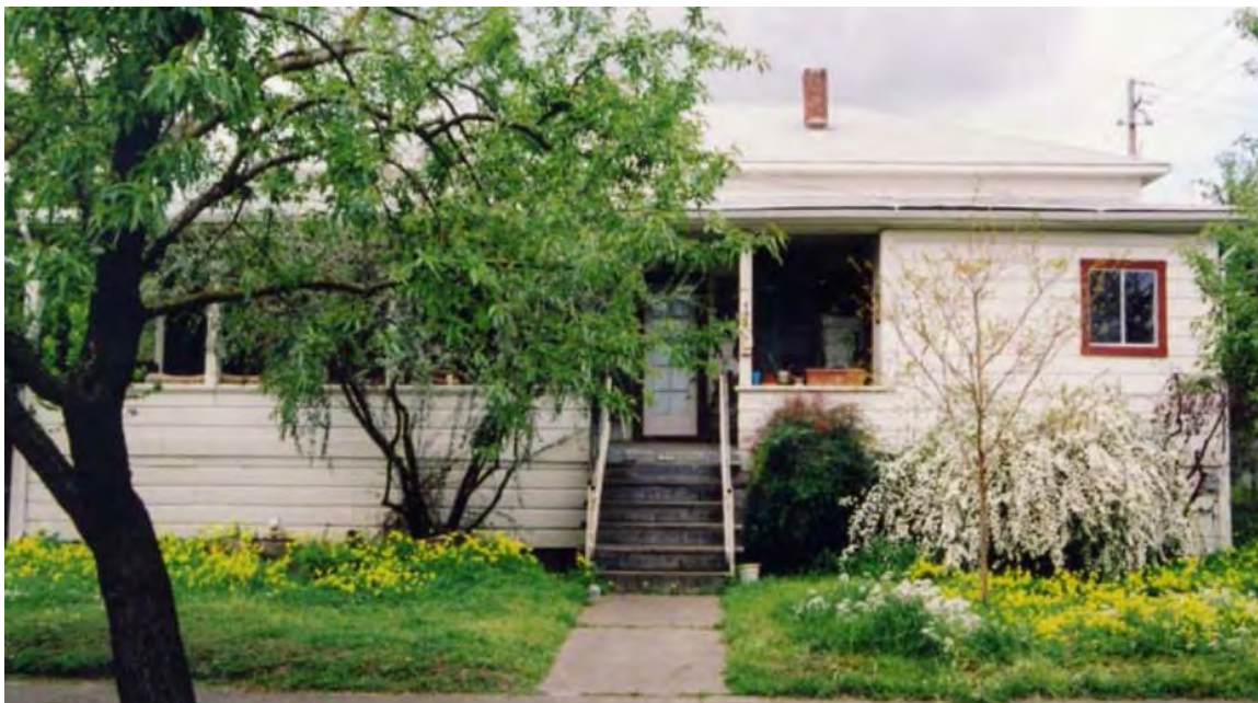
2003 Photograph; note that the right half of the original building has been removed.
