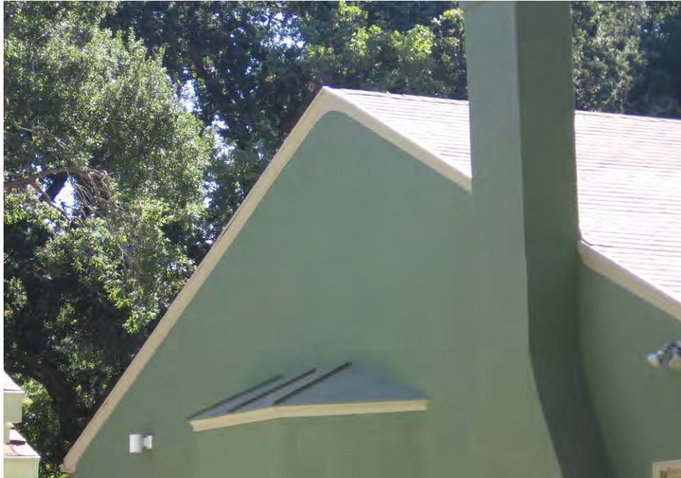
Photograph 3. Infilled window, north elevation
